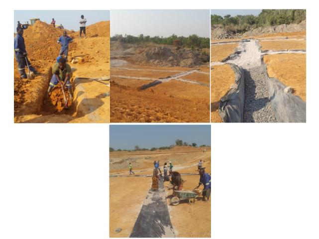
Excavation, Filling and covering of filter drains on down stream side
